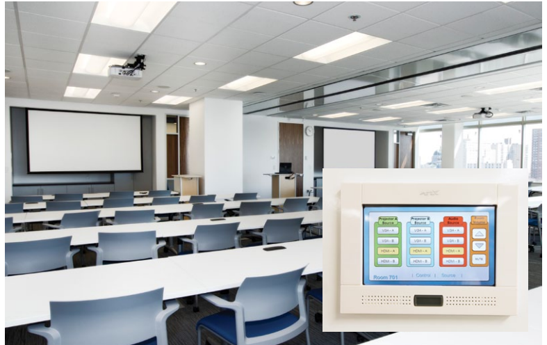
When the Skyfold wall in the dual-purpose room is open, the system is programmed to automatically feed both projectors from most analog or digital sources. When closed, the system reverts to single-room control via a wall-mounted touchpanel. Touch controls make it easy for presenters to select different content sources in the flexible Training Room.
